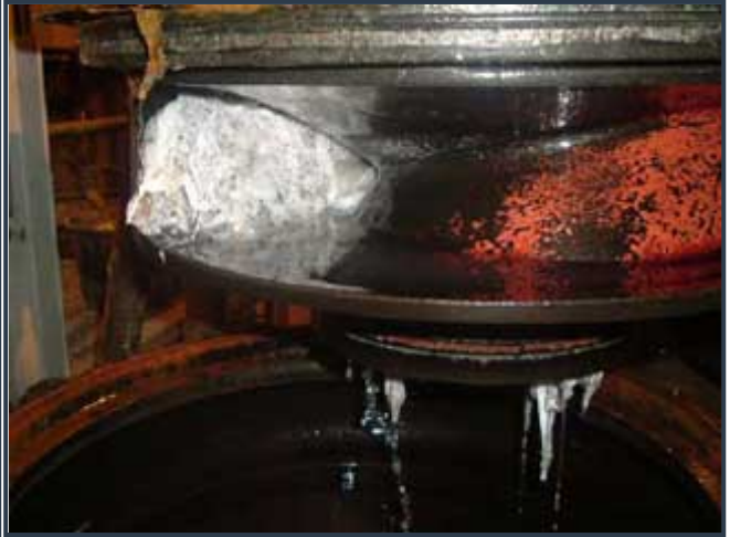
Figures 1 and 1a – Details the typical extent of a blockage in pump impellers prior to implementing new intelligent control regime.
