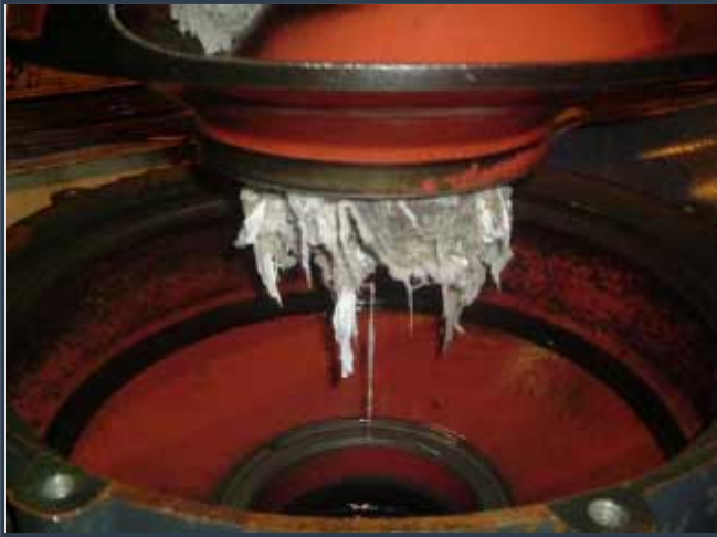
Figures 1 and 1a – Details the typical extent of a blockage in pump impellers prior to implementing new intelligent control regime.
